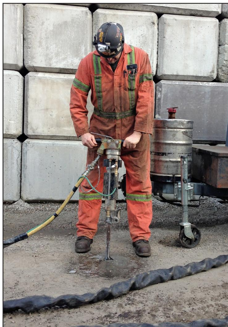
**When Winvan Paving couldn't find a sprayer attachment for its jackhammers to contain dust, it built its own. A Winvan crewmember is shown above using the dust-abatement attachment, which earned the company a VRCA workplace and health safety innovation award sponsored by WorkSafeBC**
